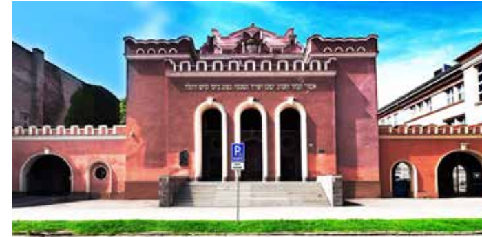
Orthox Synagogue and School (the building of Head Office ŽSR at present) Puškinova Street 3 and 5
